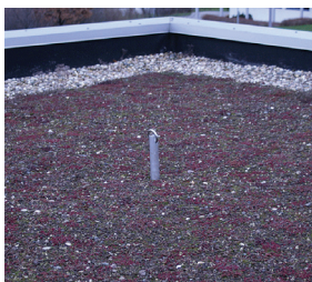
ParaSave P1 Fall Protection – installed
